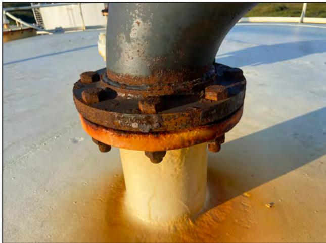
**Photo 47:** Detail view of gooseneck vent.
