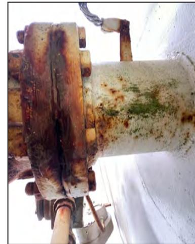
**Photo 20:** Detail view underneath blind flange (fuel transfer valve).
