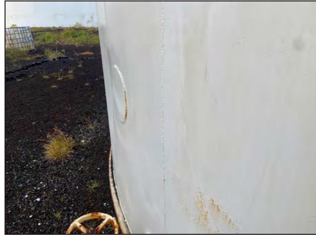
**Photo 30:** Detail view shell lap plate.
