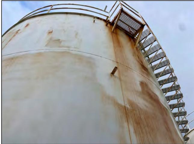
**Photo 25:** View of attachment welds and roof access (stairs).
