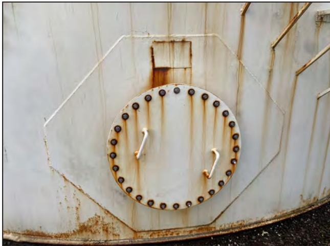
**Photo 9:** View of manway with nameplate (illegible).
