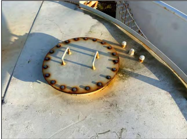
**Photo 49:** Overall view of manway and capped/plugged nipples.
