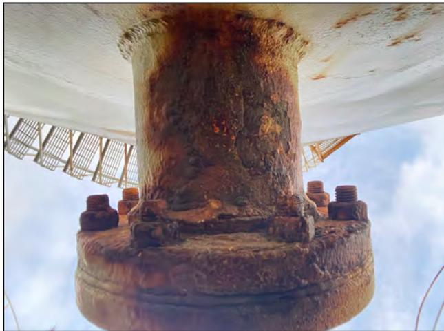
**Photo 27:** Detail view underneath blind flange (fuel transfer line).
