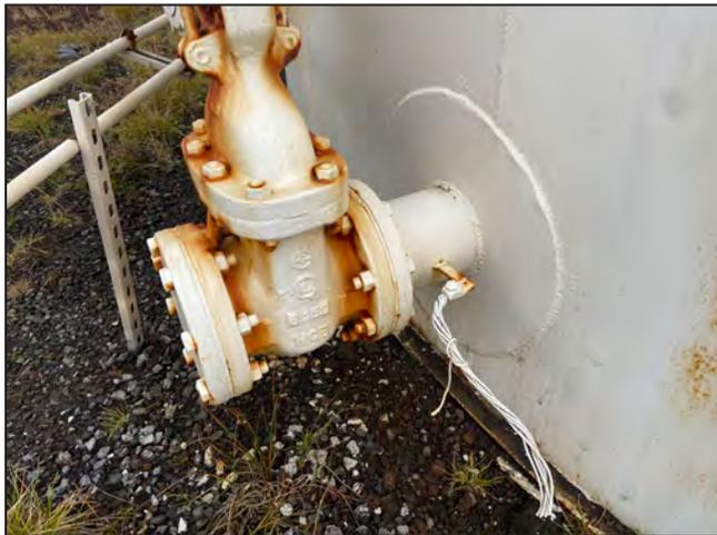
**Photo 19:** View of blind flange (fuel transfer valve).
