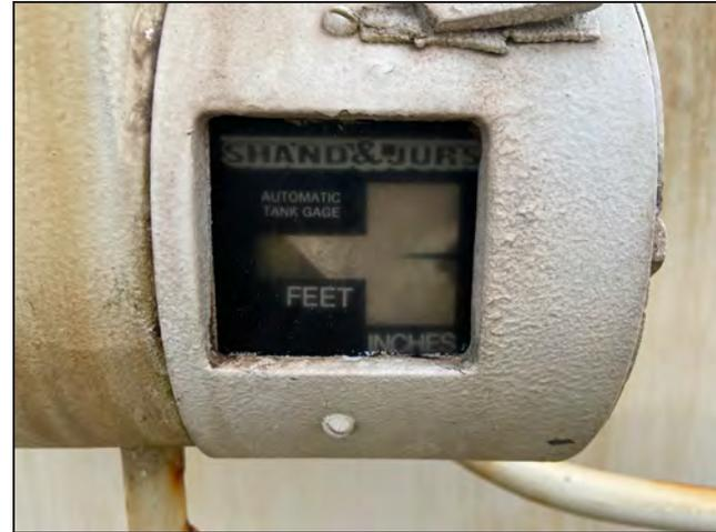
**Photo 18:** Detail view of autogauge readout.
