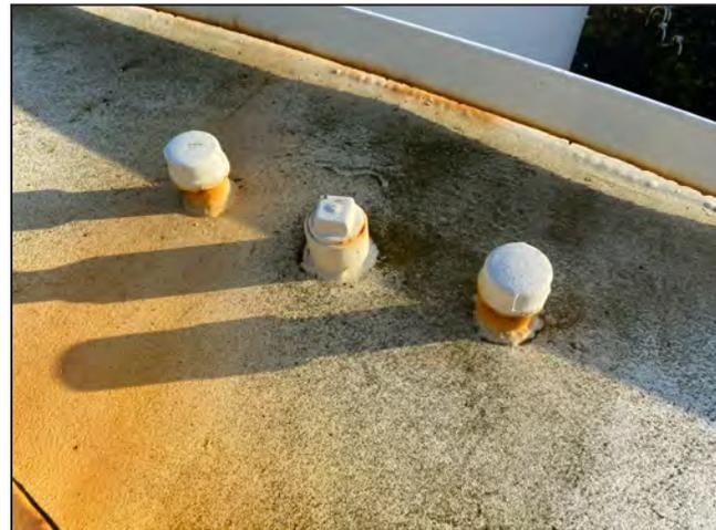
**Photo 52:** View of capped/plugged nipples.
