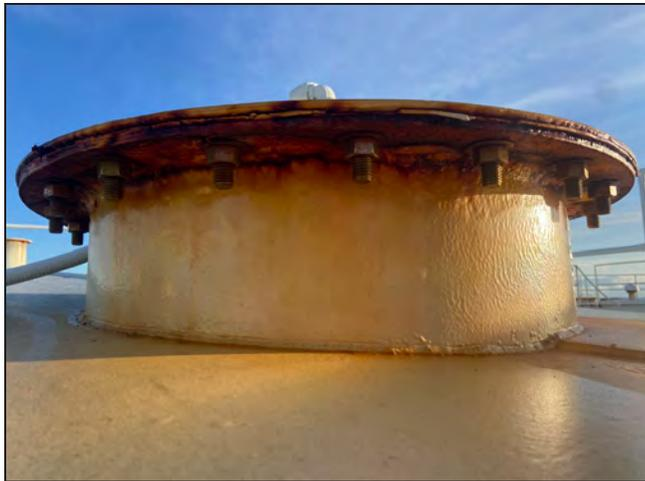
**Photo 41:** Detail view underneath manway with electronic gauging.
