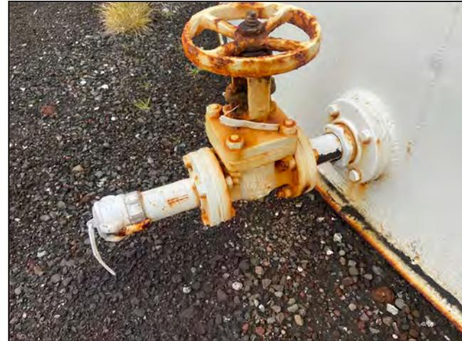
**Photo 22:** View of water draw-off nozzle (capped).
