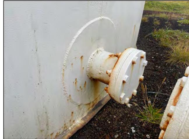
**Photo 26:** View of blind flange (fuel transfer line).
