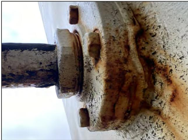
**Photo 23:** Detail view underneath water draw-off nozzle (capped).
