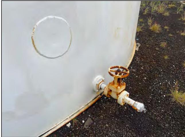
**Photo 21:** View of lap plate and water draw-off nozzle (capped).
